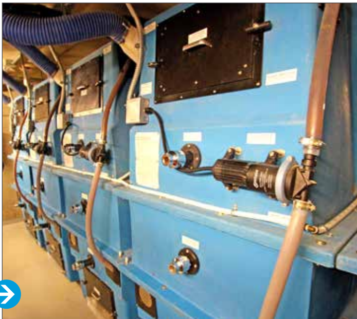
Bullitt Center also boasts 'the world's only six-story composting toilet system.' The waterless system converts solid waste into compost using aerobic digestion. (Uploaded to Flickr by Derek Severson (CC BY-NC-ND 2.0) https://creativecommons.org/licenses/by-nc-nd/2.0/legalcode .)
