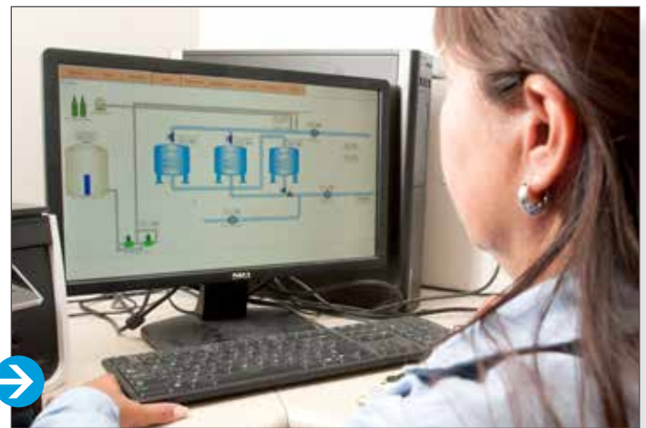
Diana Adami, Manager of the Freer, Texas Water Control Improvement District, checks the status of the Arsenic Removal System Absorber vessels using a graphical computer interface, an example of a SCADA system. (Photo by U.S. Department of Agriculture via Wikimedia Commons (CC BY 2.0) https://creativecommons.org/licenses/by/2.0/legalcode .)
