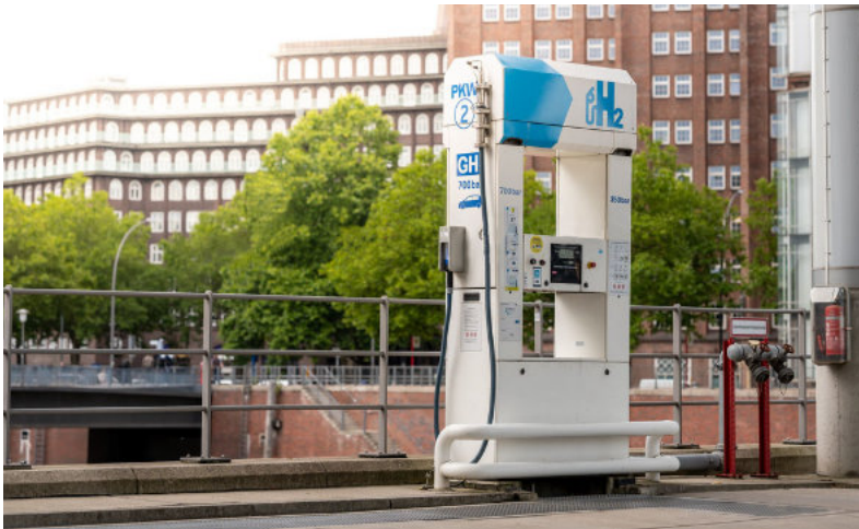
A hydrogen filling station in the center of Hamburg supplies the fuel cell buses of the Hamburger Hochbahn and fuel cell cars with hydrogen produced on site from green electricity.
